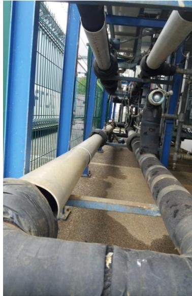
Figure 4 – Picture of the thermal grid with one of the pipe connections to the campus smart grid.
